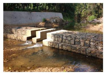
Figure 4. Gabion Check Dam
